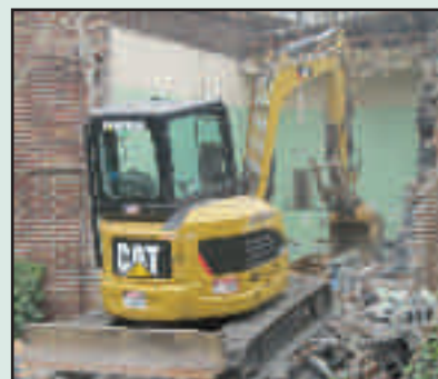
Tearing down a condemned portion of the new wing
